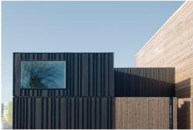
Timber and Zinc Cladding
