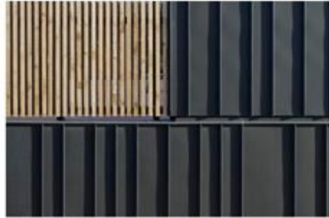
Timber and Zinc Cladding
